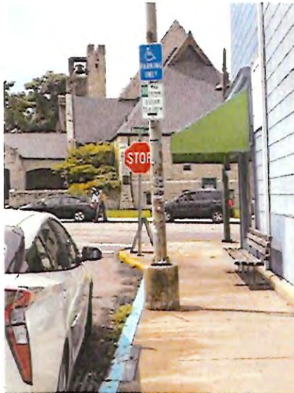
Accessible parking spot out of compliance signage is in downtown area noted
