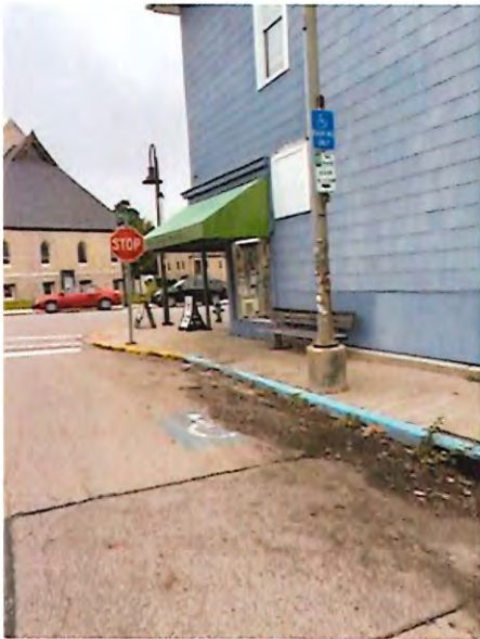
Signage is too high should be in front of accessible parking spot yellow line needs to be 2ft
